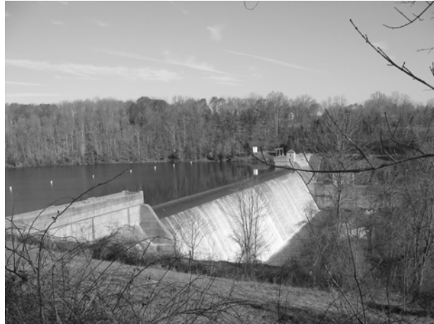
Green Lane Dam
